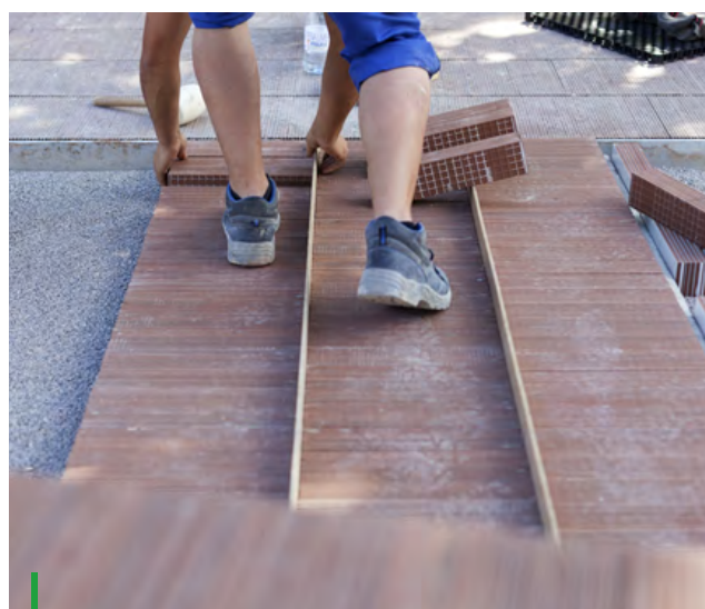
Permeable ceramic cobble installation
